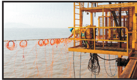
Underwater blasting operations at JNPT, Mumbai
